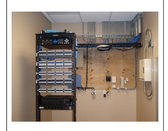
**5**: A Tier 5 Demarcation Point or Main Point of Presence where the external meets the internal interface.
