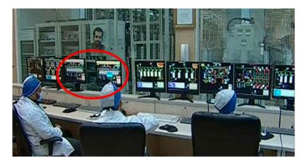
The control room of the above-ground Pilot Fuel Enrichment Plant (PFEP) as of February 2012, with operators sitting in front of SCADA screens. The two displays highlighted in red run the monitoring application for the Cascade Protection System that is discussed in-depth in this document.
